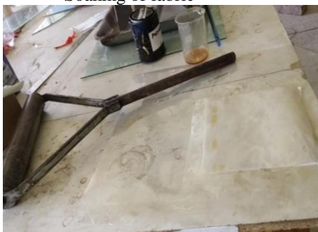
Preparation for PU coating (direct coating)
